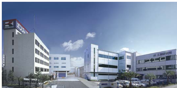
Head office and factory
